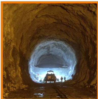
View of benching operation in Diversion Tunnel in Pakal Dul HEP
