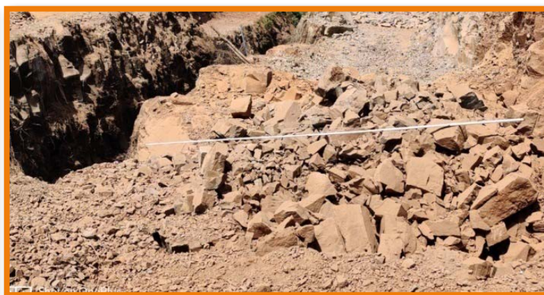
View of blast and throw of post blast rock materials (Throw controlled within blasting area) at Bordave and Shirsewane Cutting sites in Konkan Railway
