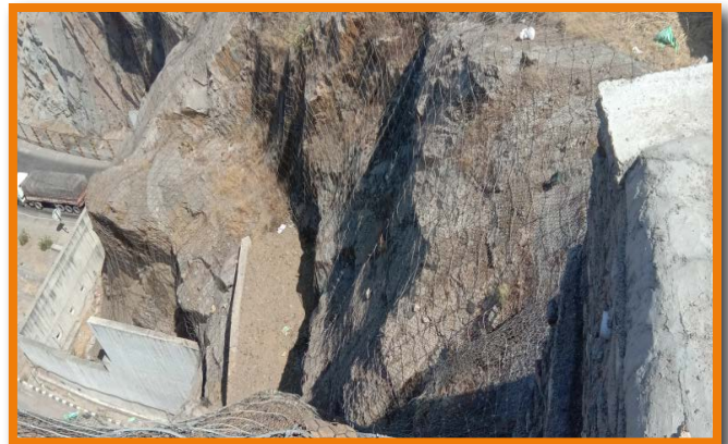
Photo 5 (a) Kinematic feasibility at Portal slope; (b) stabilized section with rock bolt and DT mesh
