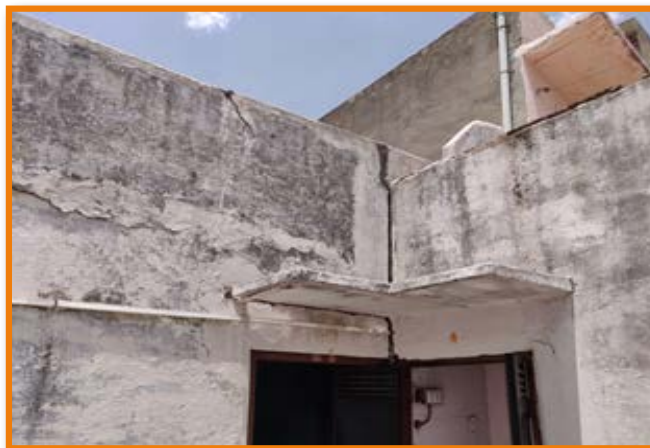
Photo: Cracks in Houses of Pur Village
