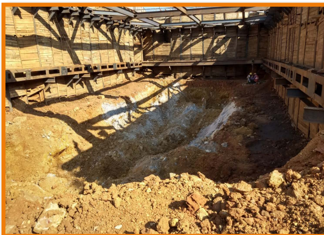
View of blast face in track hopper area of 2 x 660 MW Obra-C Thermal Power Plant
