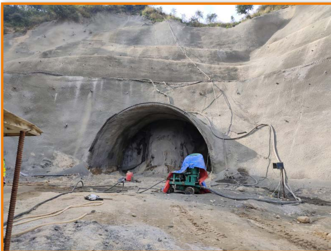
Fig.3: False portal of T2P2 with supported slopes
