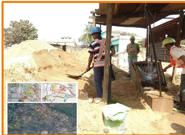
Fig. 3. Blind backfilling in Talcher area, MCL
