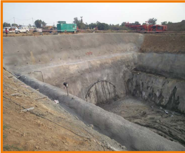
Fig. 4: Unstabilized slope, drainage and tunnel face
