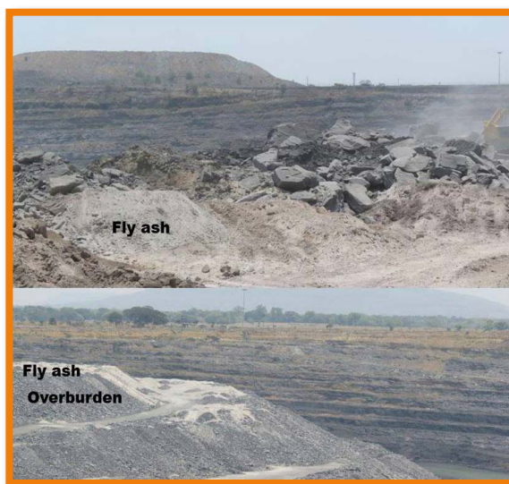
Fig.1. Ash filling in opencast mines
