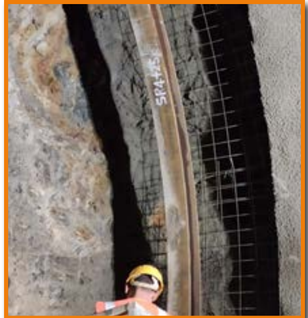
Installation of rib in Adit 3
