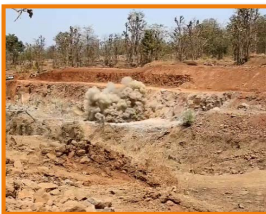
View of blast and throw of post blast rock materials (Throw controlled within blasting area) at Bordave and Shirsewane Cutting sites in Konkan Railway
