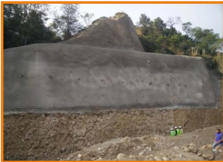
Fig.1: Slope above tunnel portal T1P2 under excavation
