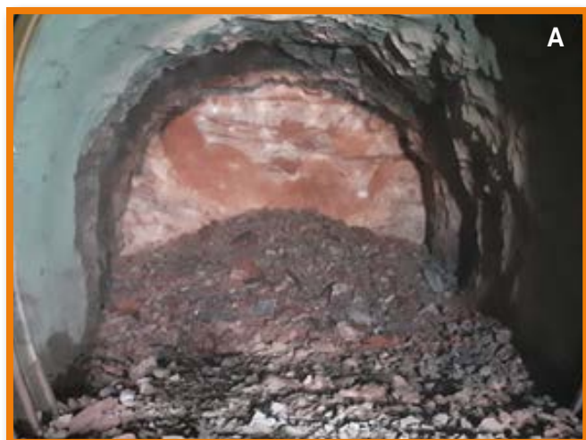
Figure A: Blasting operation and blast vibration monitoring at Jamalpur
