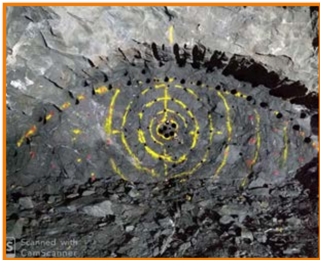
Blasting of shot-hole present in the 1 st ring
