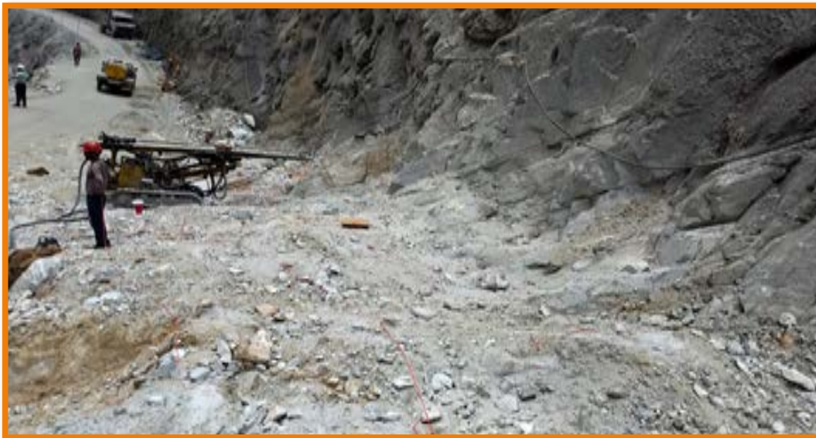
Photo 1: Charged face of Open Bench for DAM Cutting
