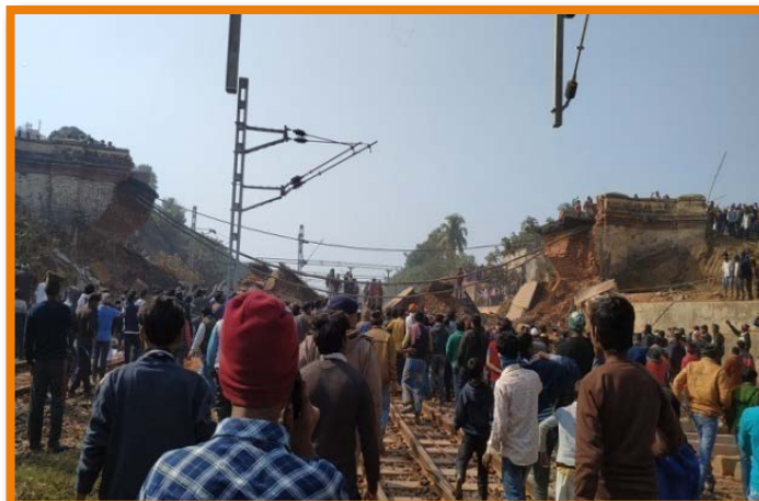
Views of before and after demolition of ROB No. 91 near Pirpainti Station, Bihar using controlled blasting
