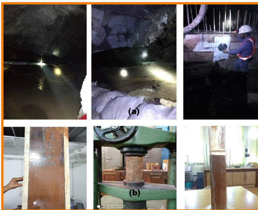
Fig. 4. Backfilling at Mahagiri mines (a) Backfill pouring and stable backfilled stope (b) Experimentations with OB
