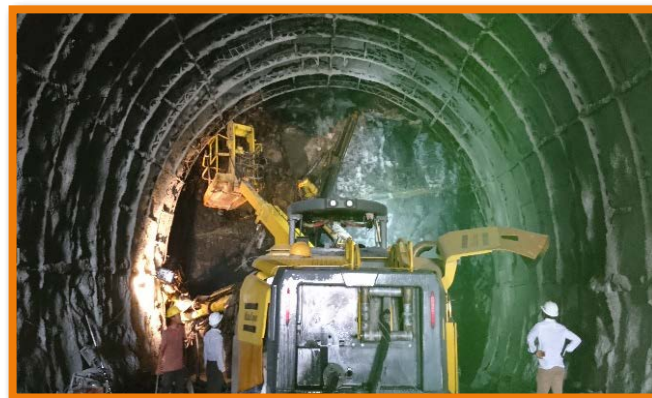
Fig.2: Primary support using shotcrete, rock bolts, wire mesh and lattice girders
