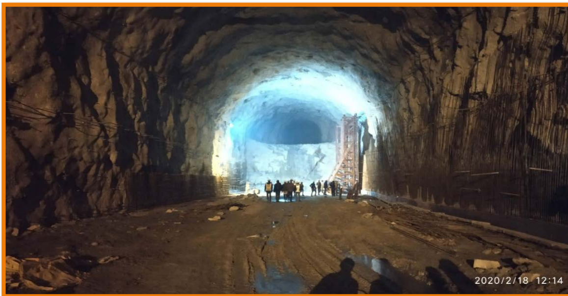
Photo 2: Benching in Desilting Chamber (DC 3)
