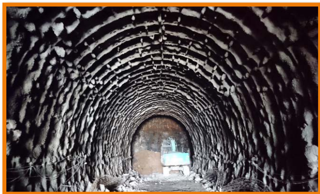
Fig.1: Railway tunnel with soil in crown and weathered basalt in bottom of the face
