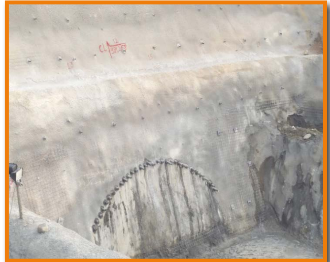
Fig. 5: Face with roof-pipes at T4P1
